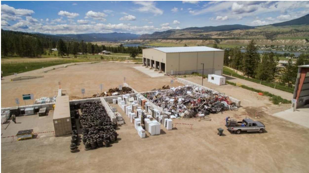
Figure 3: TNRD South Thompson (Pritchard) Eco-Depot 9
