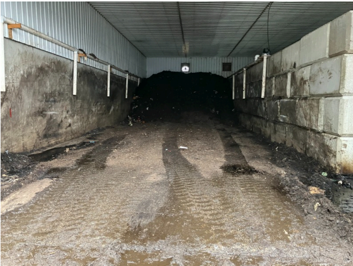
Photo 2. Composting facility located on concrete to prevent the release of leachate into the environment.
