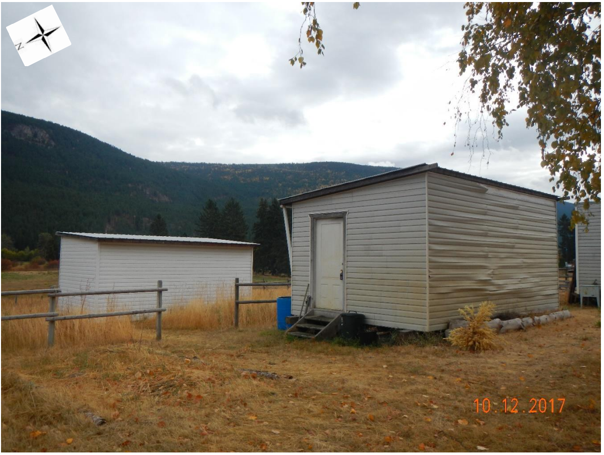
Facing southeast at the accessory buildings
