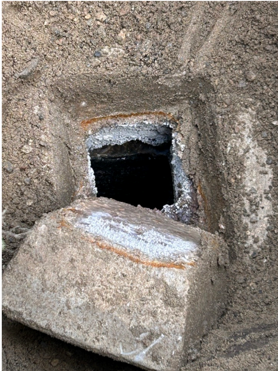
Photo 4. Outlet access hatch.
