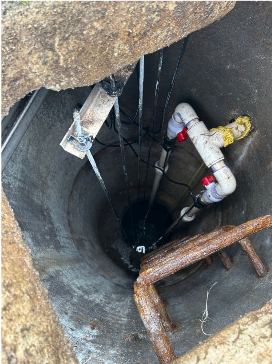
Photo 6. Inside the pump chamber. Duplex pumps/high level alarms.
