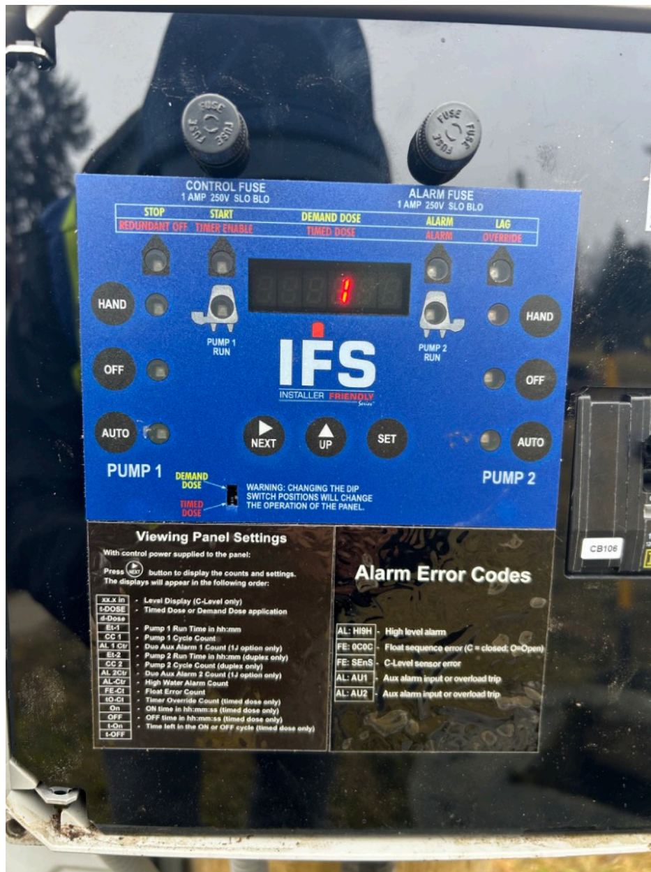
Photo 7. Rhombus control panel. Pump A: 3200 doses. Pump B :3250 doses. Average of 253h of run time each. Audible and visual alarm operating normally.
