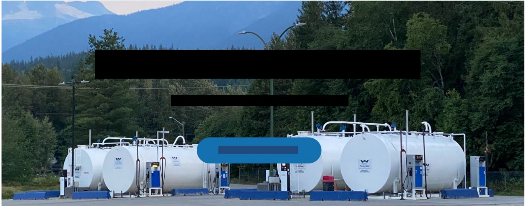
Example of cardlock fuel service station with above ground tanks
