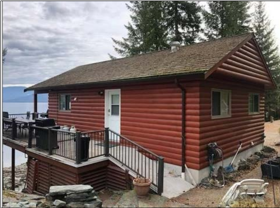
Photo of Existing Boathouse with suite facing east submitted by agent
