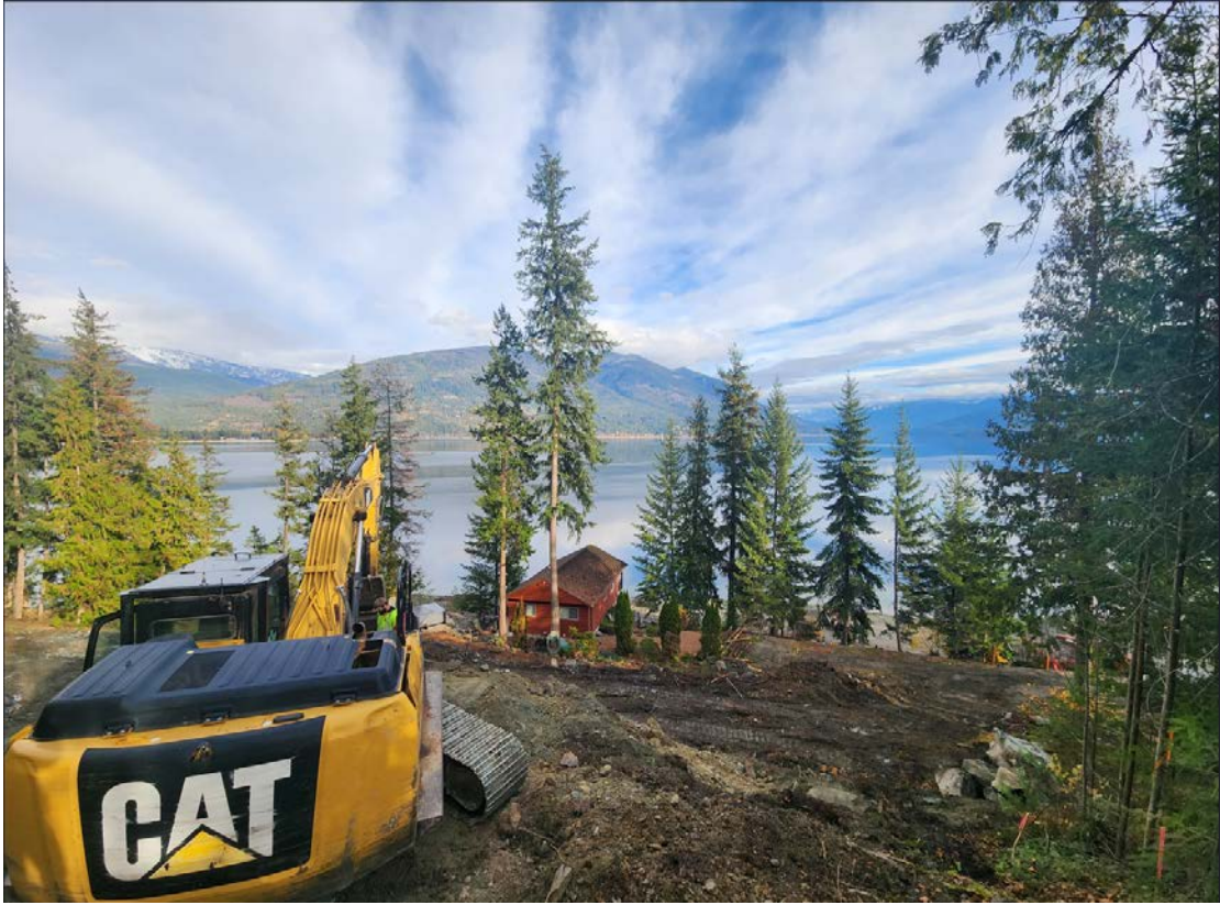
Photos of proposed location of single detached dwelling facing northeast
