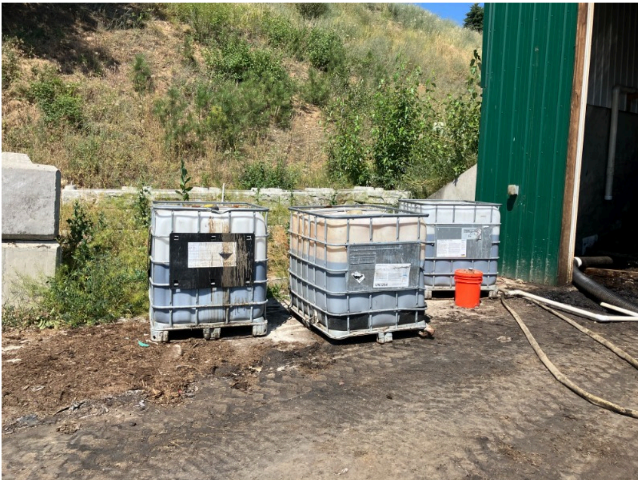
Photo 4. 4500L leachate collection system Facility recycles the leachate back into the composting process.
