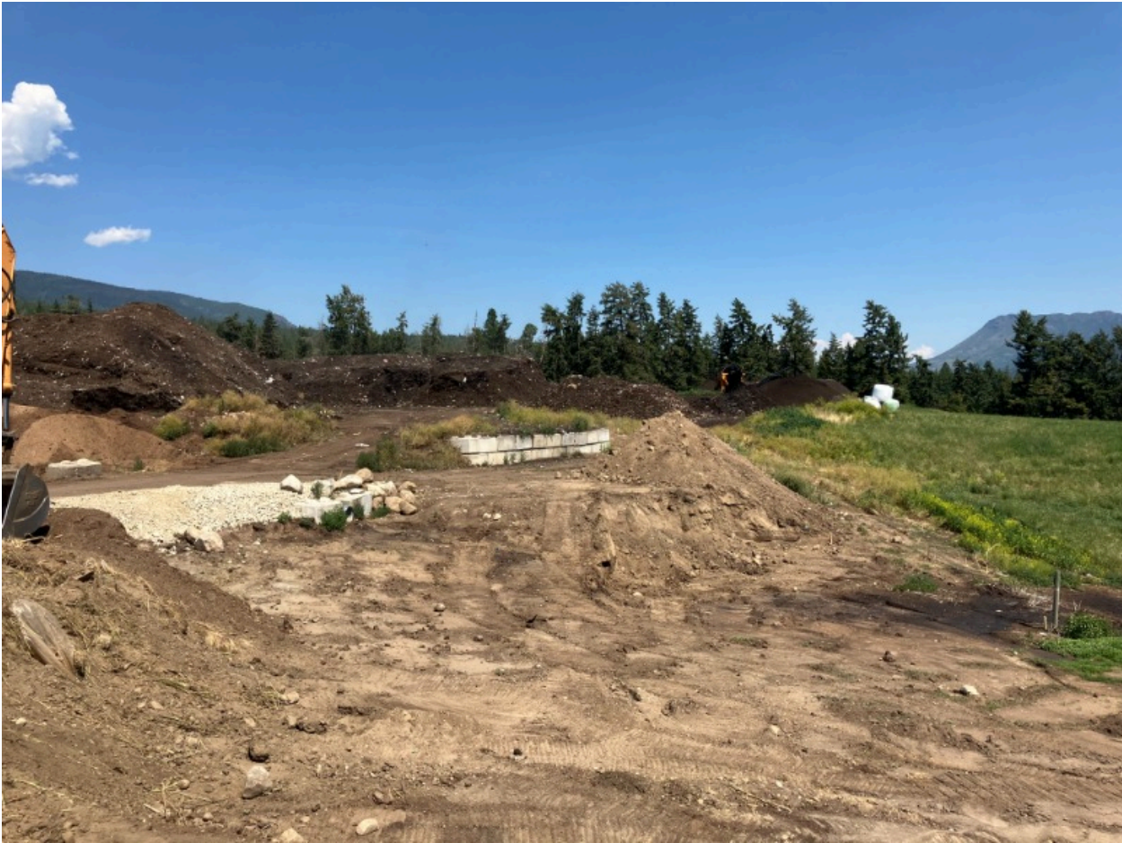
Photo 5. The storage area at the Facility did not have a roof, cover or a prepared surface designed to prevent the surface collection of water around the base of organic matter.
