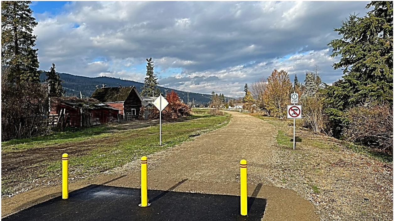
Enderby-Splatsin Pilot Section – entrance bollards and signage (completed November 2023)
