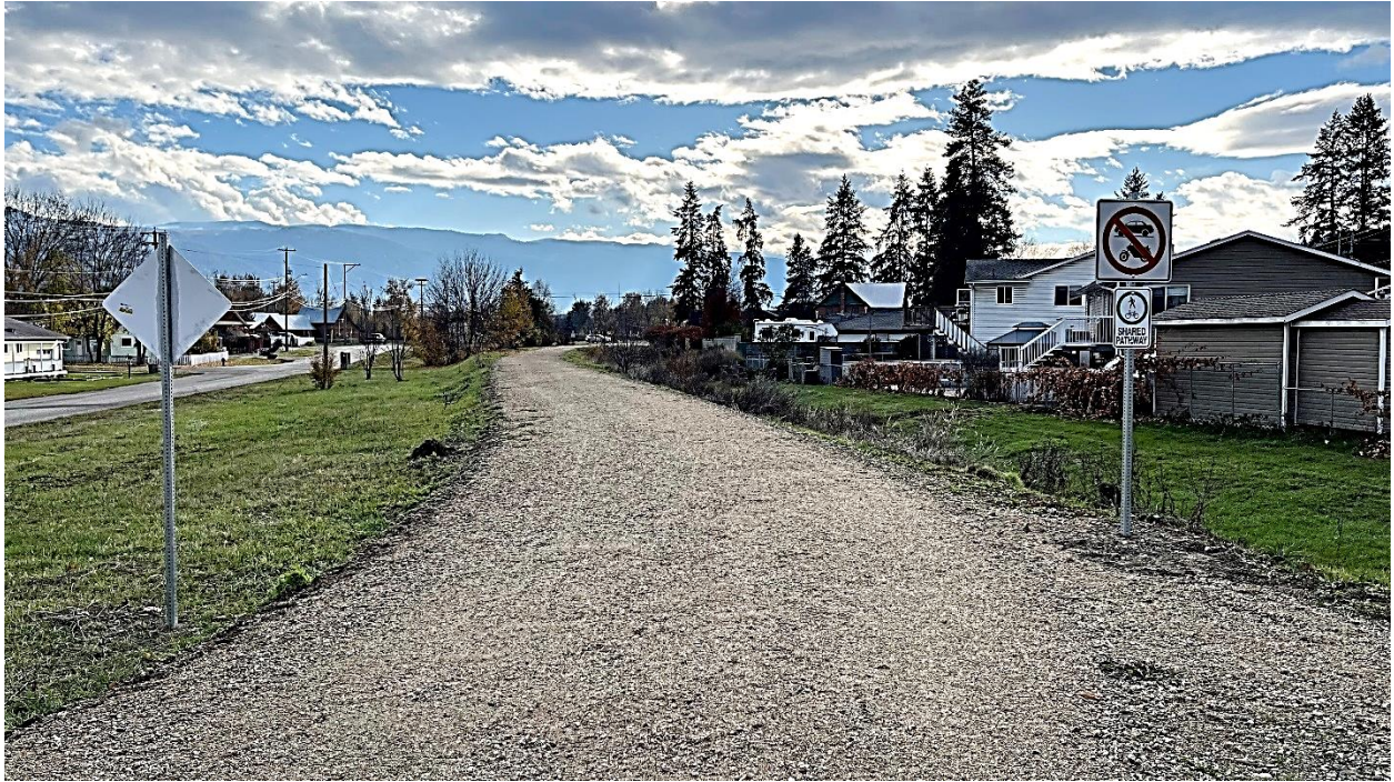
Enderby-Splatsin Pilot Section – newly packed aggregate surfacing (completed November 2023)
