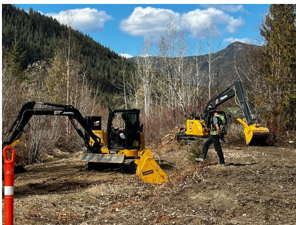
Preparation of staging area at Folland Road.
