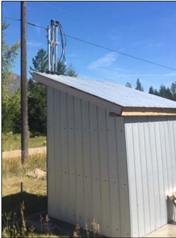
Photo of pumphouse building
