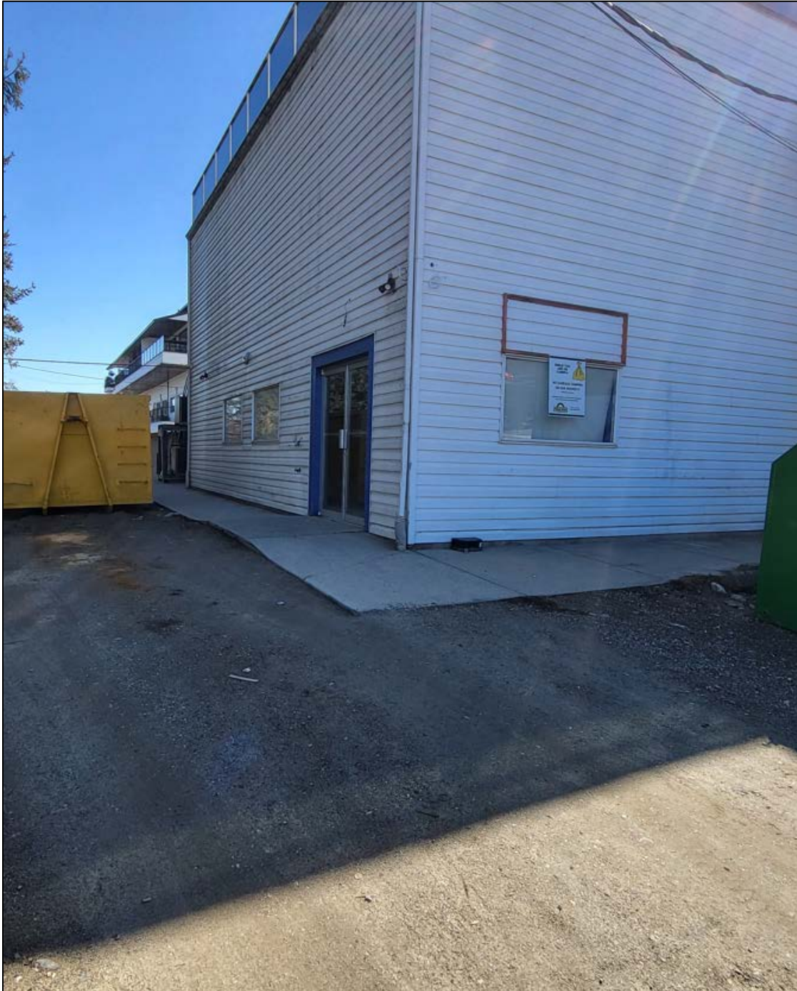
Rear of Building where Bottle Recycling Drop Off Facility will be
