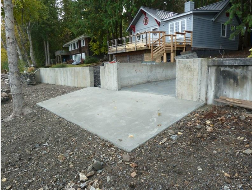
Photo 3. A failing section of rock/concrete retaining wall in front of the cabin and a disintegrating boathouse floor were recently replaced with new concrete. Both the retaining wall and boathouse are above the high water mark of Shuswap Lake (348.7 m).
