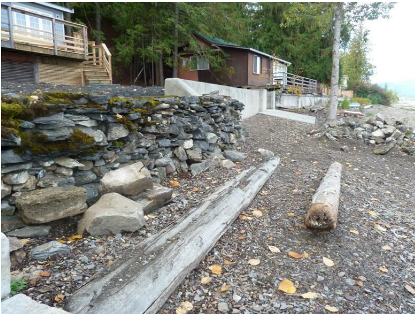
Photo 4. A failing section of retaining wall (1.1 m high by 8.2 m long) was replaced with concrete and stepped ~0.4 m further back from the high water mark of Shuswap Lake.
