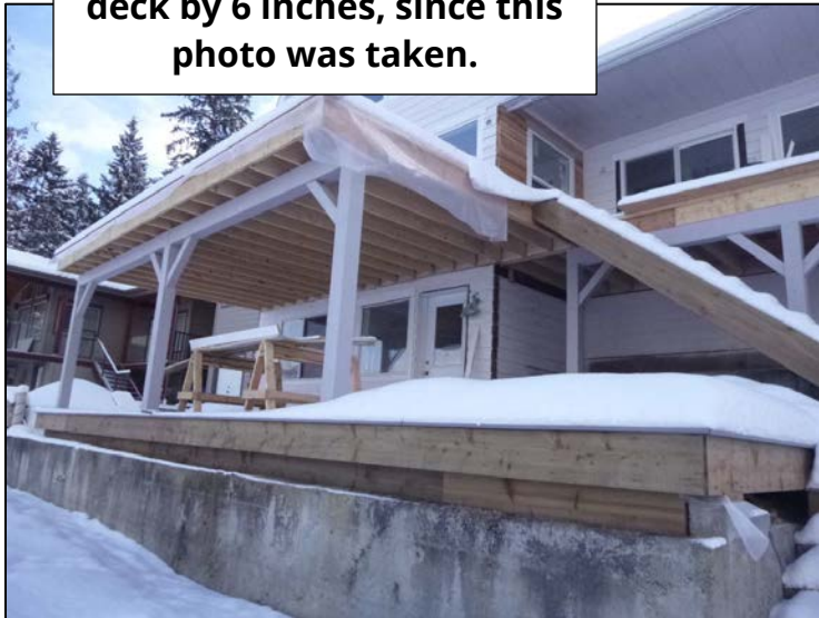
Photo 4: Recent photo submitted by the applicant showing that the deck has been cutback 0.15 m (6 inches).
