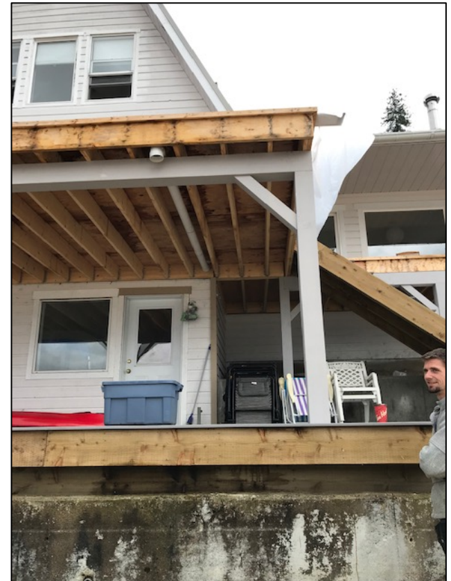
Photo 4: Recent photo submitted by the applicant showing that the deck has been cutback 0.15 m (6 inches).
