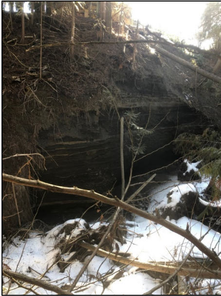
Photo 4: Looking across at undercut bank and high erosion at Civic address 2819.
