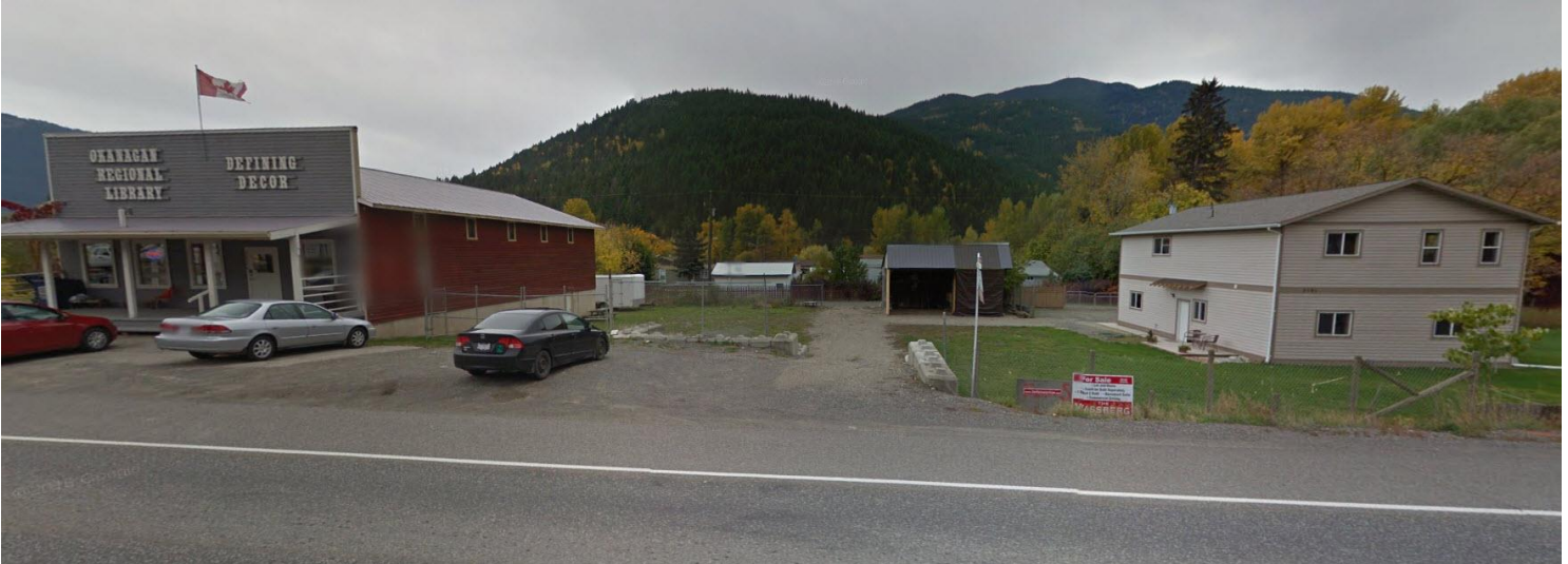
View of subject property to the far right, vacant lots in the middle, and Okanagan Regional Library to the far left
