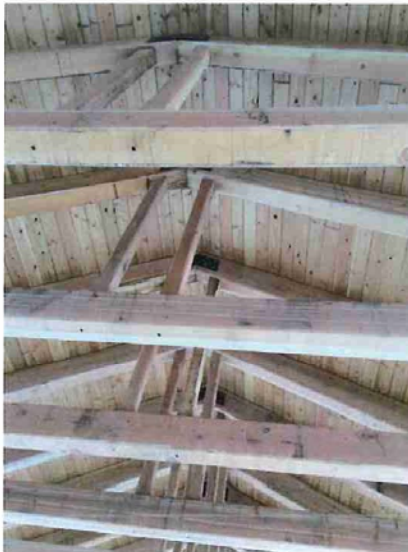
Photograph 9. Roof structure – untreated cedar - January 2016
