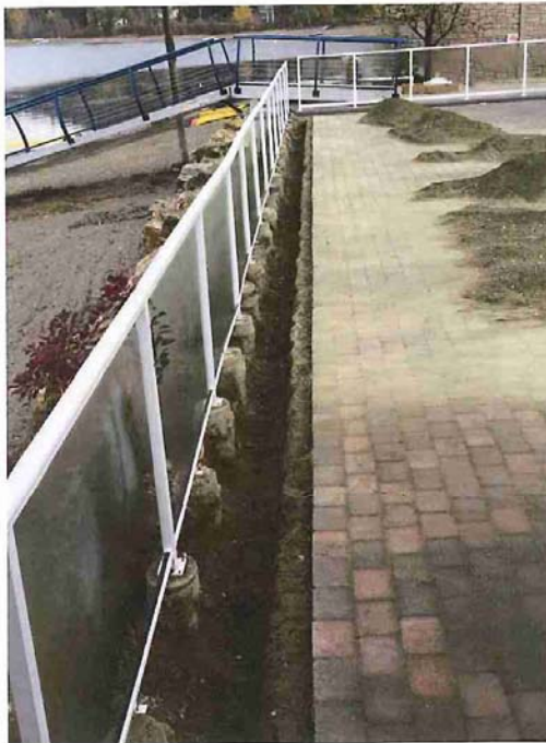
Photograph 3. Patio railing footings are revealed – Fall 2015
