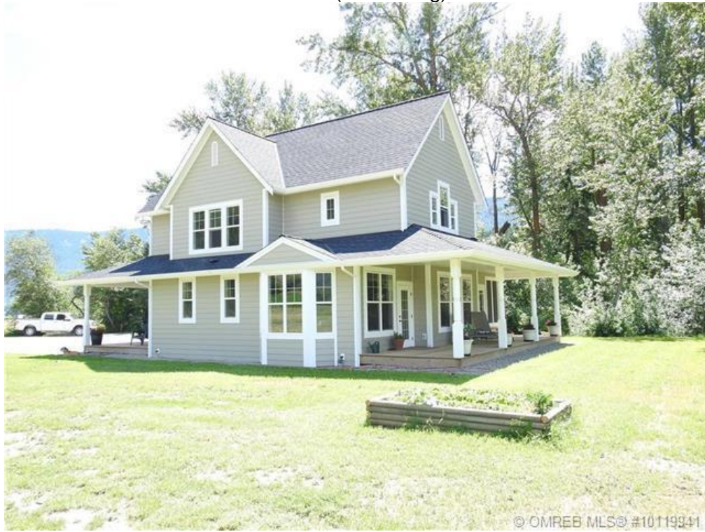
Facing south at the "new" single family dwelling
