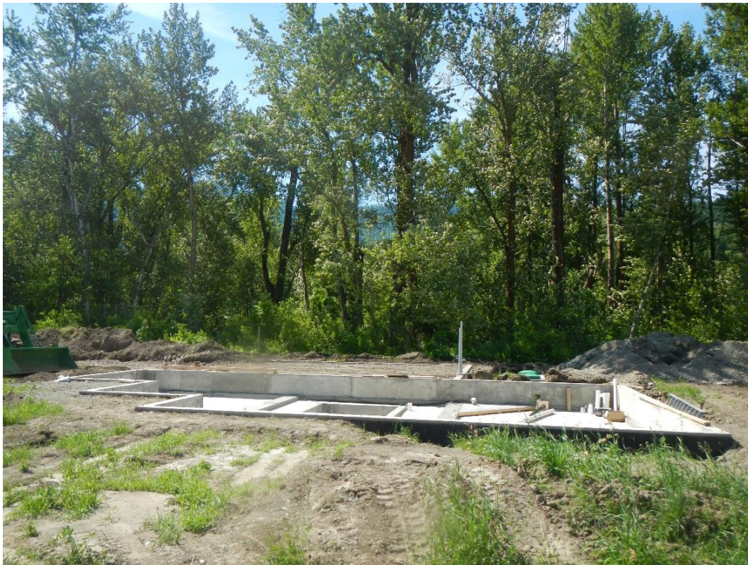
Facing south at the foundation of the "new" single family dwelling
