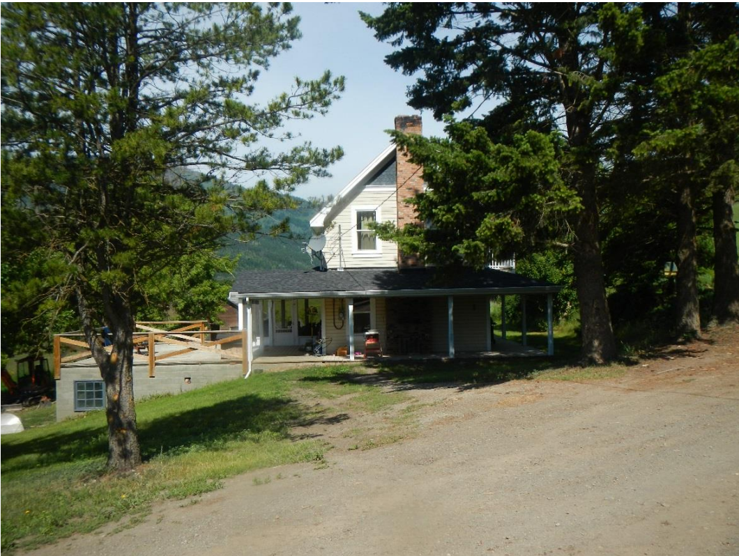
Facing northwest at the "old" single family dwelling
