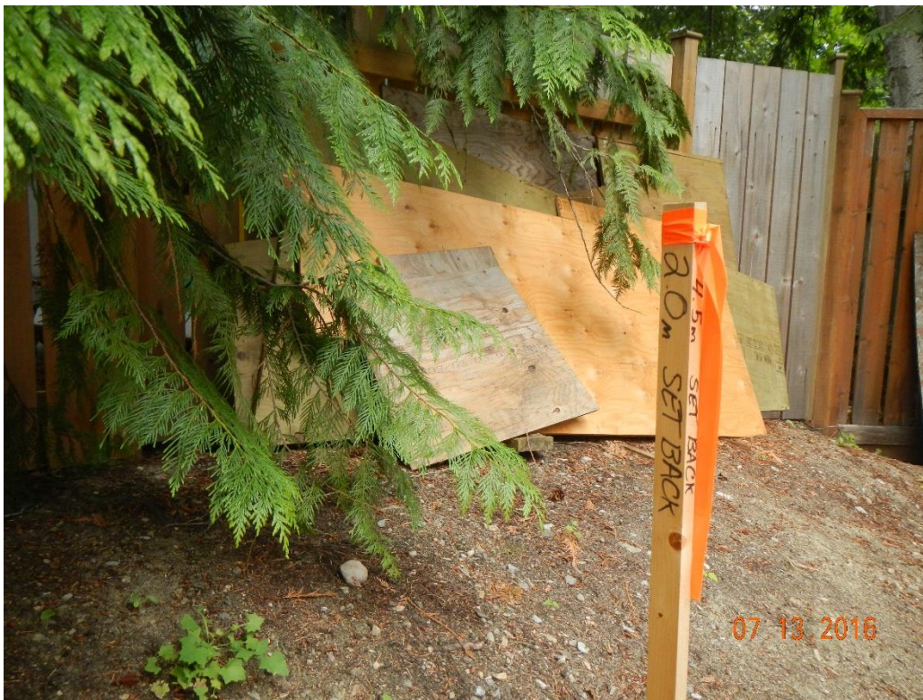
Facing west at one of the surveyor's stakes indicating the setbacks
