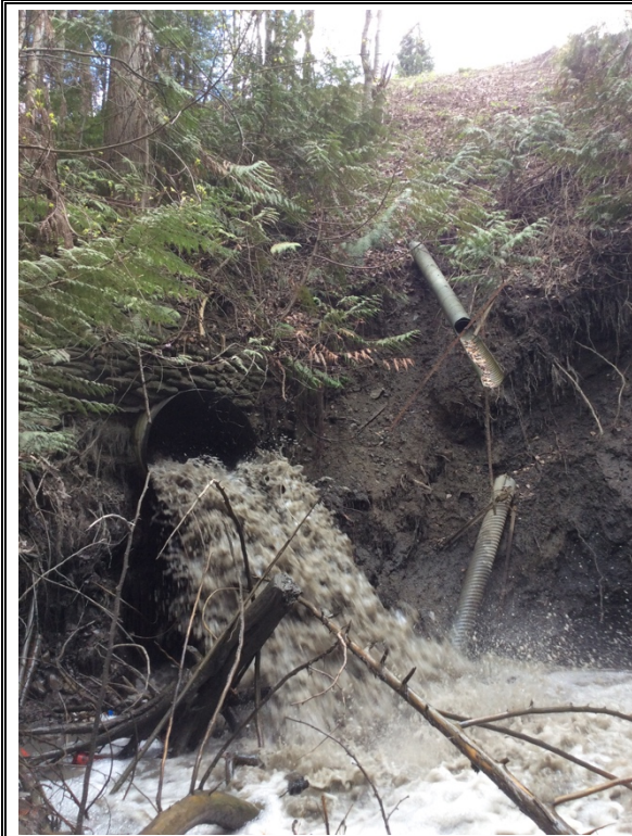
Photo 7 – View of culvert outlet (1200 mm diameter) in Highway 1. Note the scour in the embankment to the immediate right. [May 1, 2018]
