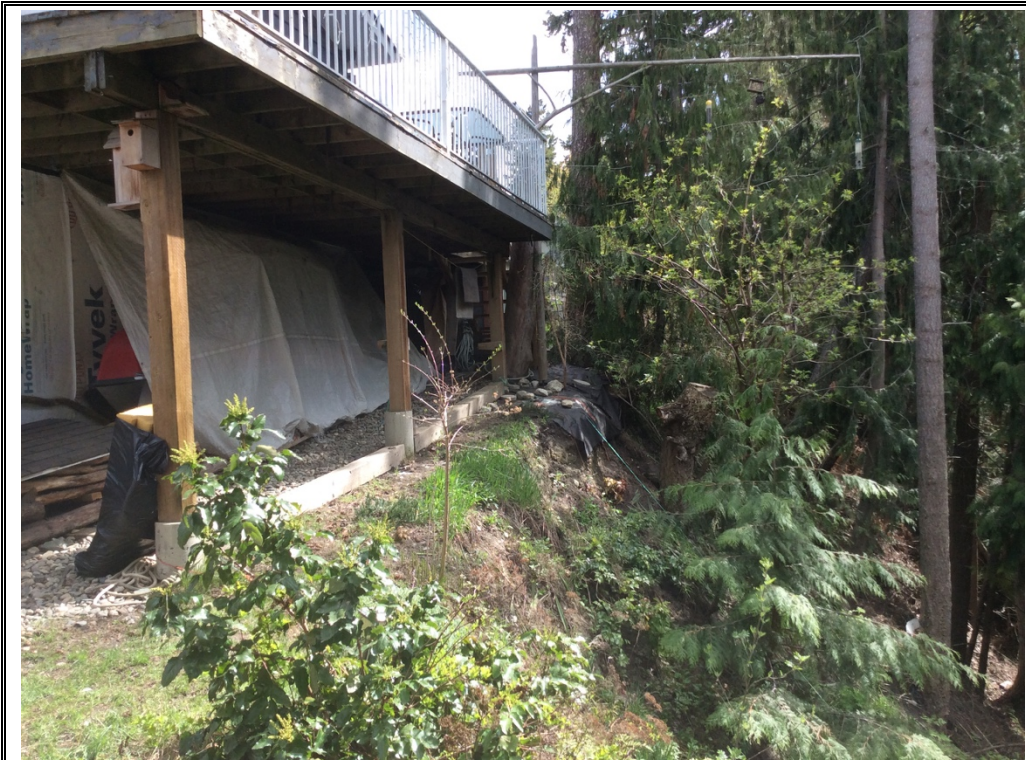
Photo 11 – 2809 Caen Road: view looking upstream along the gully crest at the very steep slope below the elevated deck. The house is about 3 m back from the crest. A shallow debris slide occurred below this area (see Photo 12). [May 7, 2018]
