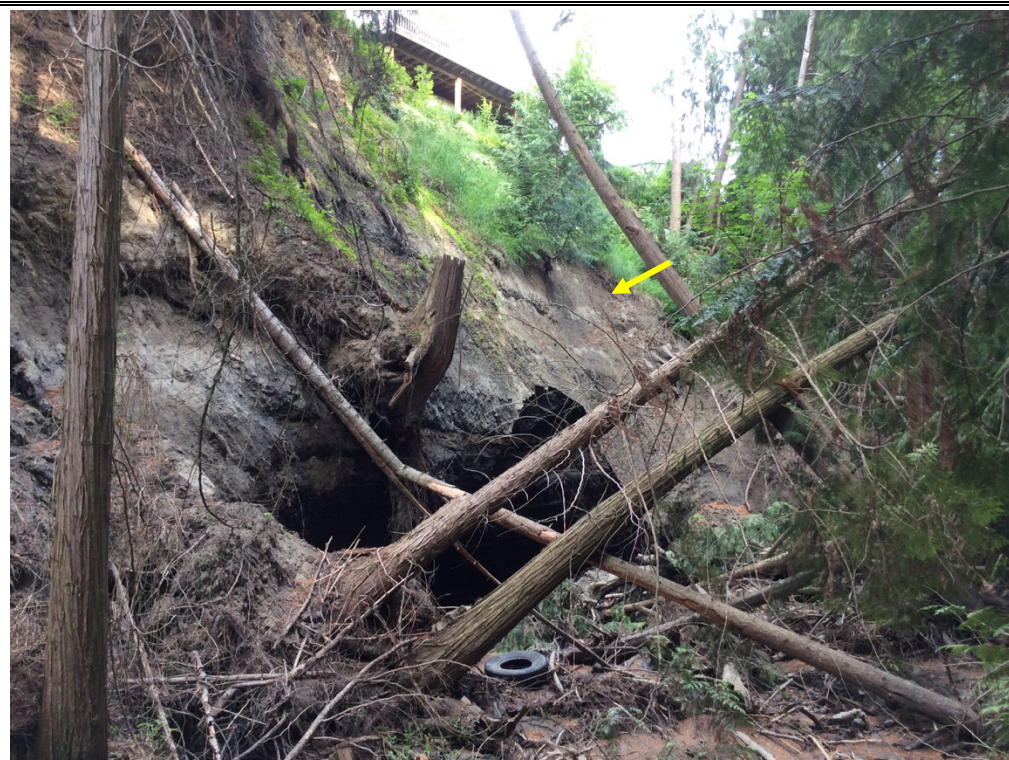
Photo 12 – 2809 Caen Road: view looking upstream at the bank instability. The elevated deck is visible in the background. A small debris slide (arrow) that occurred early in May 2018 is shown with the arrow. [May 26, 2018]
