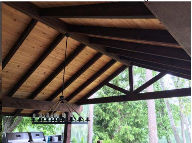
Timber Roof Rafters
