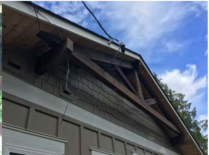
Timber Beams and Rafters supported on Timber Cantilevered Beams through wall
