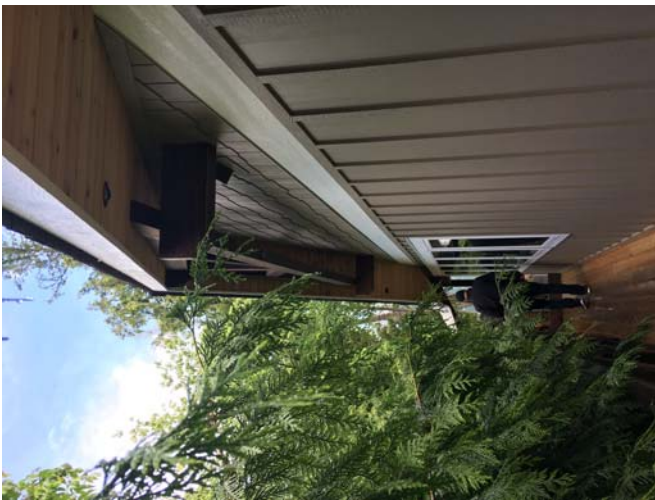
Timber Beams and Rafters supported on Timber Cantilevered Beams through wall
