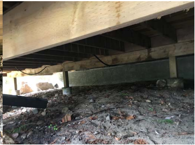
4 x 4 Post Supporting 2 ply 2 x 8 Beam
