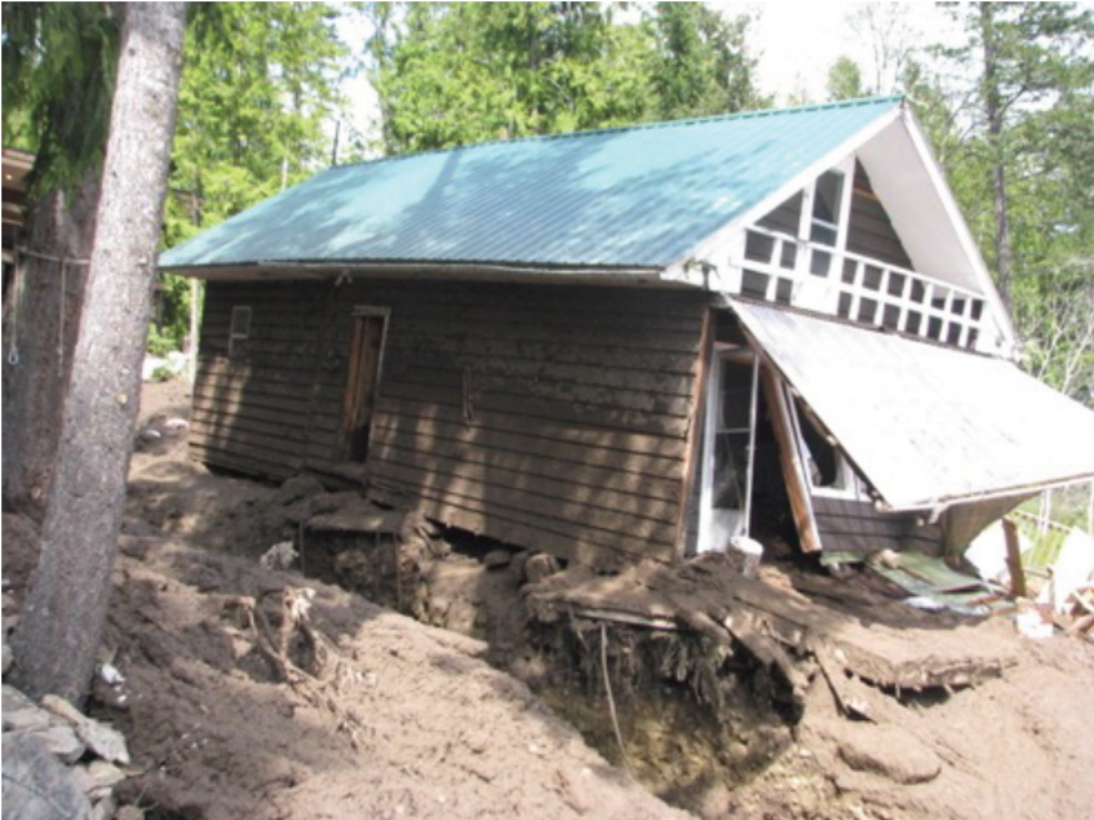
Photo 23 – View northeast of the ancillary residence on the 5932 Sunnybrae – Canoe Point Road. Debris passed through and may have been displaced the building. The creek now passes along the west side of the structure (foreground).
