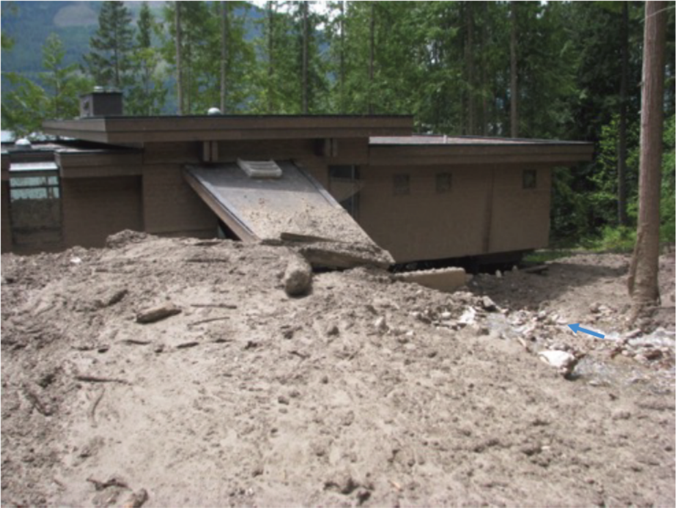
Photo 21 – View downstream of the primary residence on the 5932 Sunnybrae – Canoe Point Road, showing debris piled up against the north wall. The debris flow passed through and around the residence, and the stream (blue arrow) now flows under the structure.
