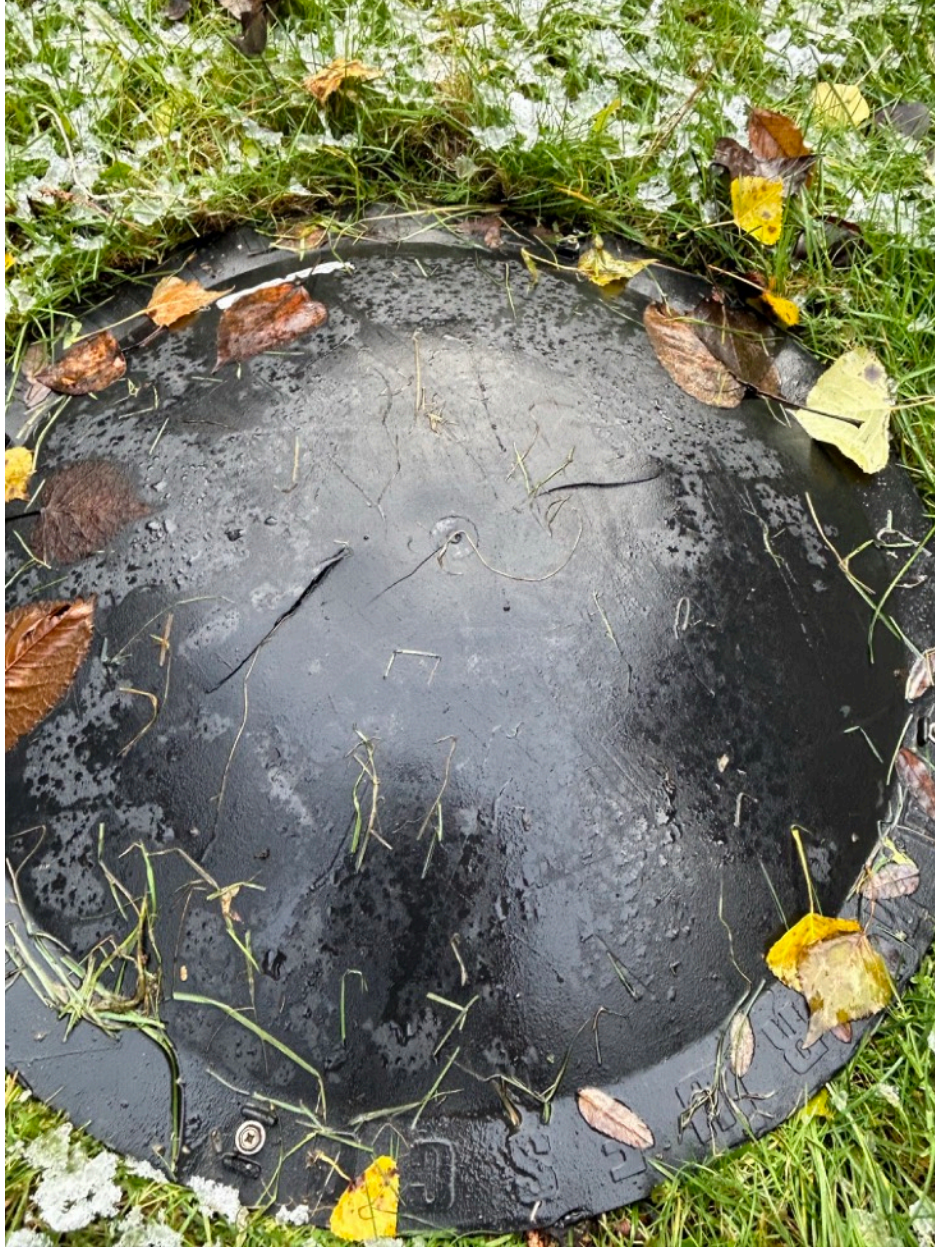
Photo 3. Main access lid (to be replaced).
