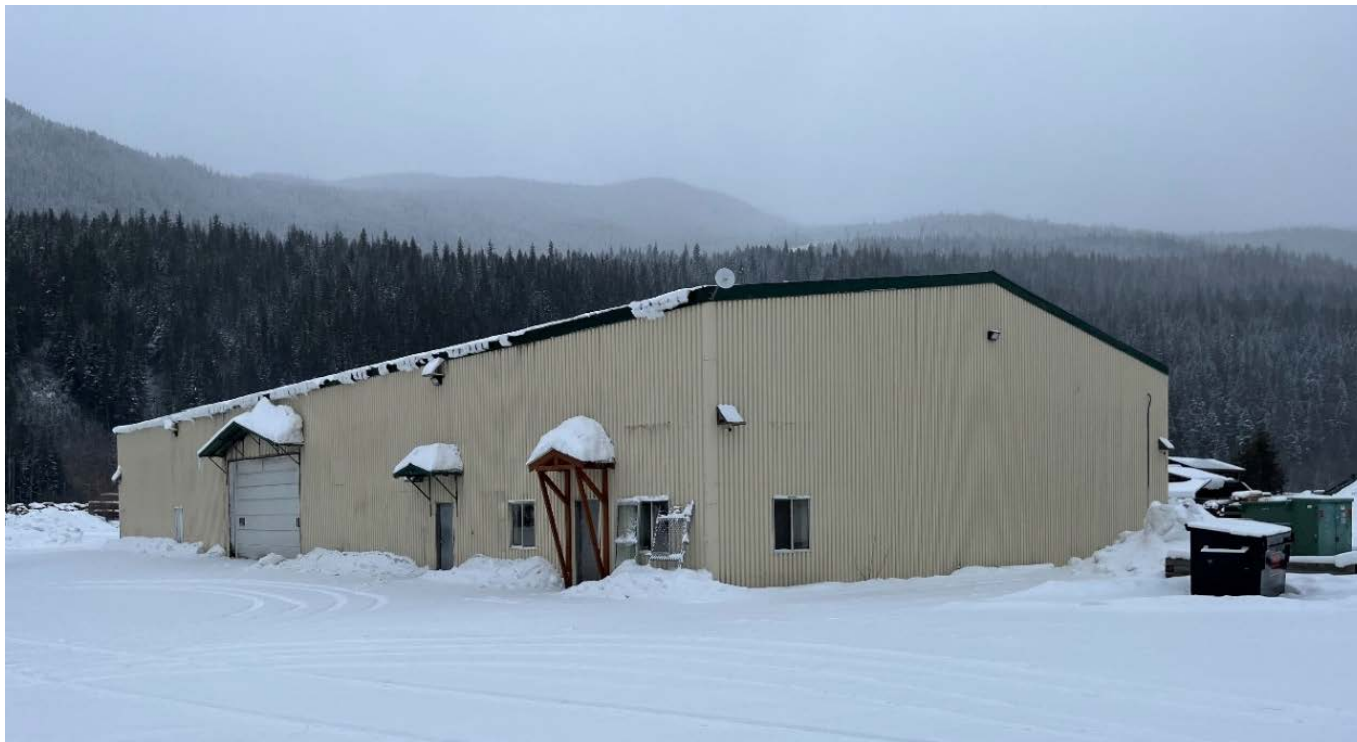
Existing Commercial Storage Building
