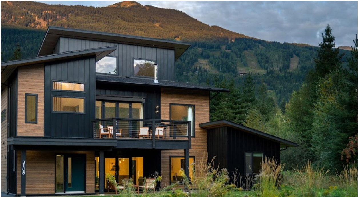
Photo – Lodge (Capow House)
