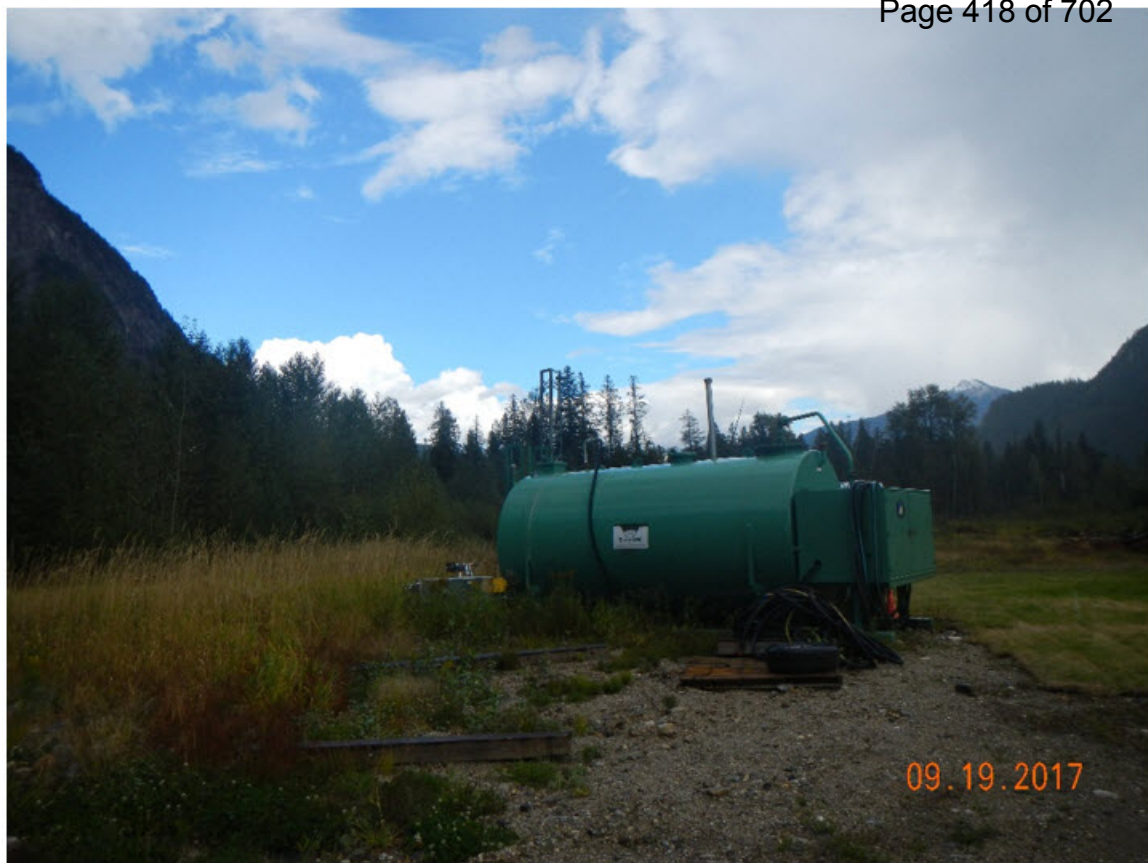
Fuel storage tank for helicopter refueling
