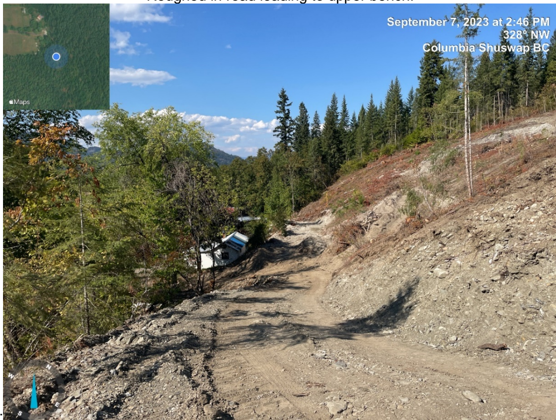
Roughed in road leading to upper bench:
