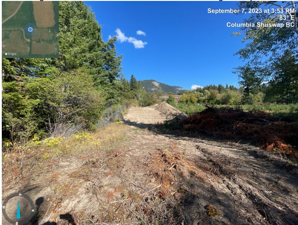
Roughed in access road from Colton Road – through ALR portion:
