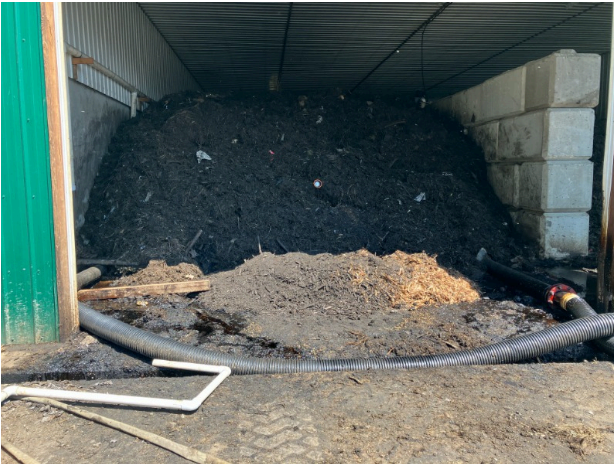
Photo 1. Processing and curing areas of the composting facility, located on concrete and covered with a leachate collection system.
