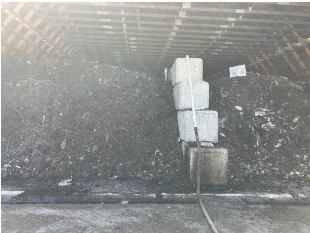
Photo 2. Receiving, processing and curing areas of the composting facility are located on concrete and covered.
