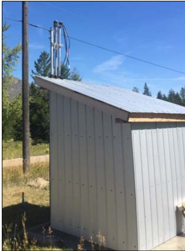
Photo of pumphouse building
