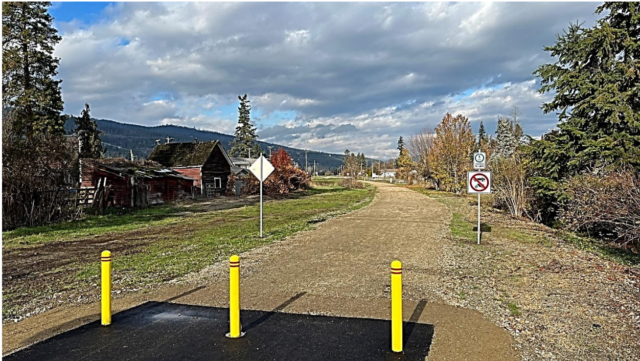
Enderby-Splatsin Pilot Section – entrance bollards and signage (completed November 2023)
