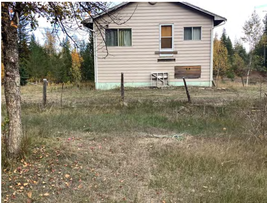
Photo 2. View of abandoned house in the disturbed yard area of the subject property along the CSRD mapped stream. Photo looking east.
