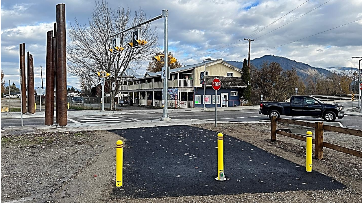
Enderby-Splatsin Pilot Section – Cliff Avenue Pedestrian activated crosswalk.
