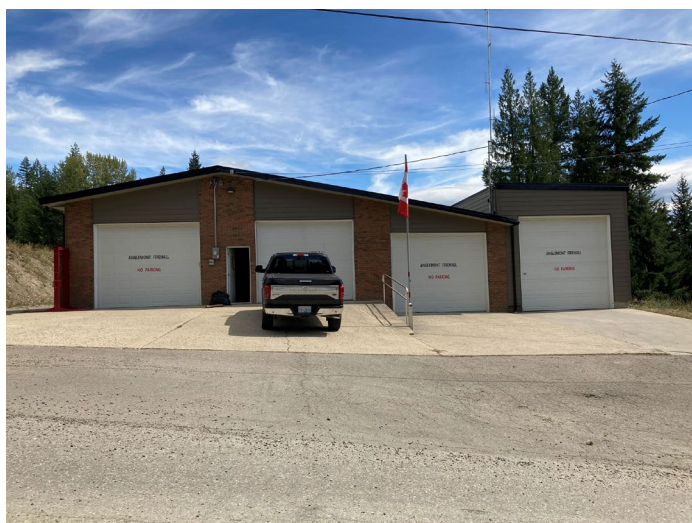
Figure 13: Anglemont fire hall
