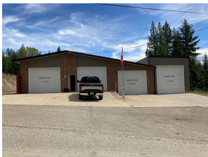
Figure 13: Anglemont fire hall
