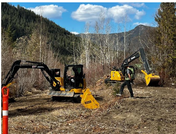
Preparation of staging area at Folland Road.
