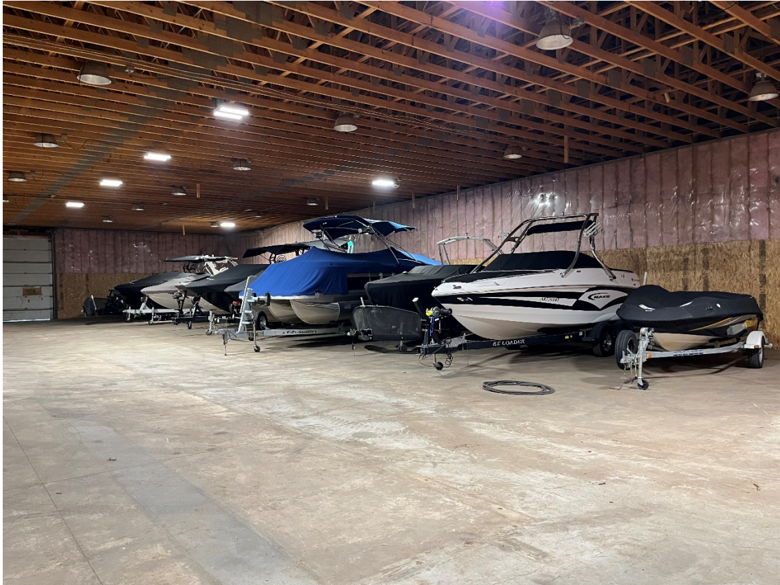
Existing storage building
