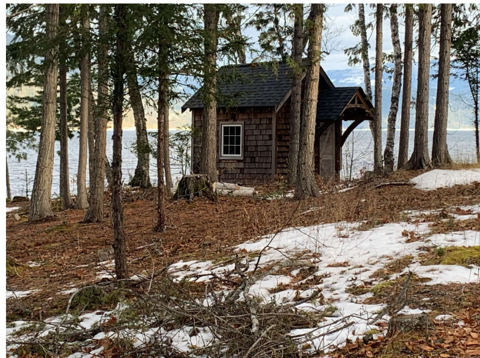
Label Photo 6: North-east view of existing historic shed (January 2023).
