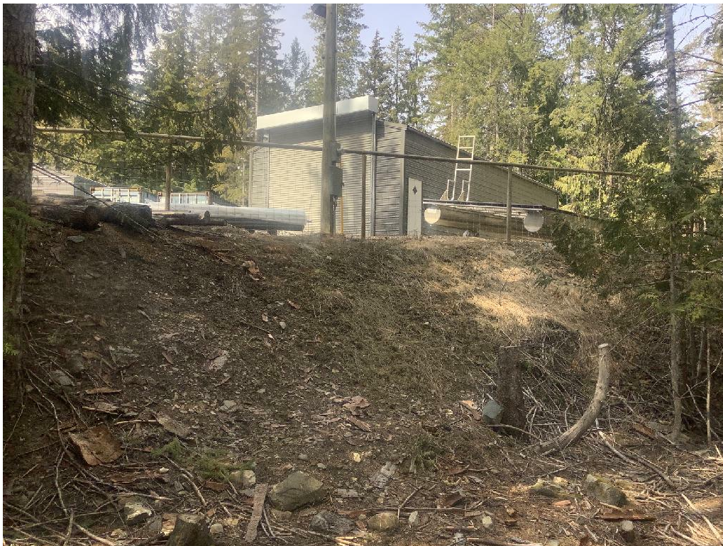
Photo 10 The moderate to moderately steep slopes of the fill surrounding the shop structures in the southern portion of the Remainder Lot, looking southwest.
