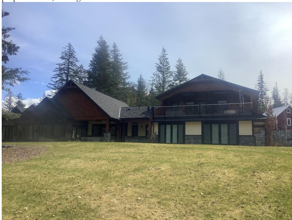
Photo 8 Existing residential structure on the Remainder Lot, looking south.
