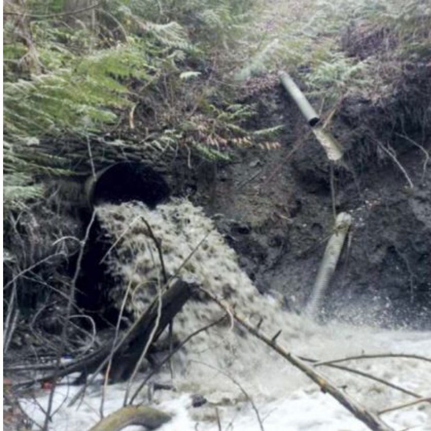
Culvert at Highway 1 May 2017
