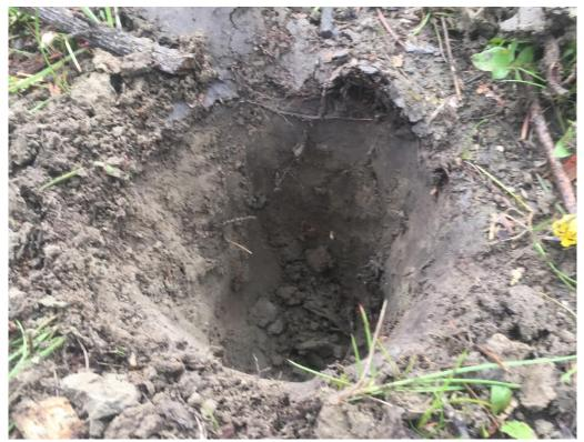
Photo 3 Soil profile on the property consisting of firm SILT some fine sand
