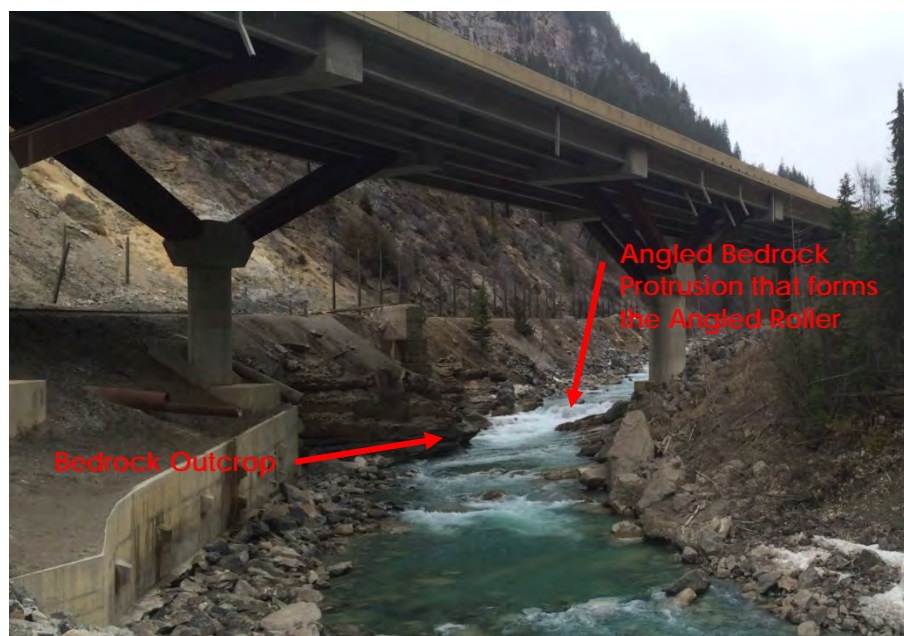
Figure 9 - Looking upstream at Angled Roller and Bedrock Outcrop (Image courtesy of Ryan Johanneson April 13, 2016)
