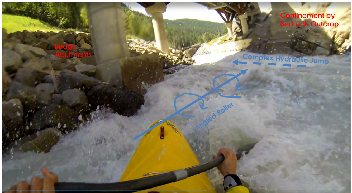
Figure 7 - Hazardous Hydraulic Conditions Approaching Five Mile Bridge Looking Downstream (Image courtesy of Mikkel St. John-Duncan)
