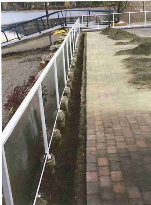
Photograph 3. Patio railing footings are revealed – Fall 2015
