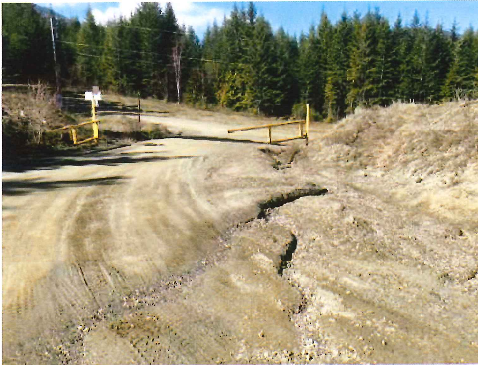
Photo 3 Erosion from surface runoff on the access road at Gate 1, looking west.
