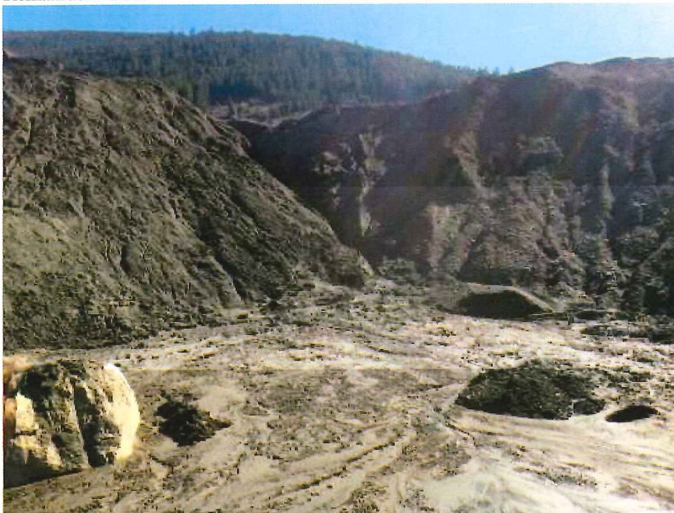
Photo 8 Runoff down coming from the upper pit to the middle pit causing a slurry of deposition, looking east.
