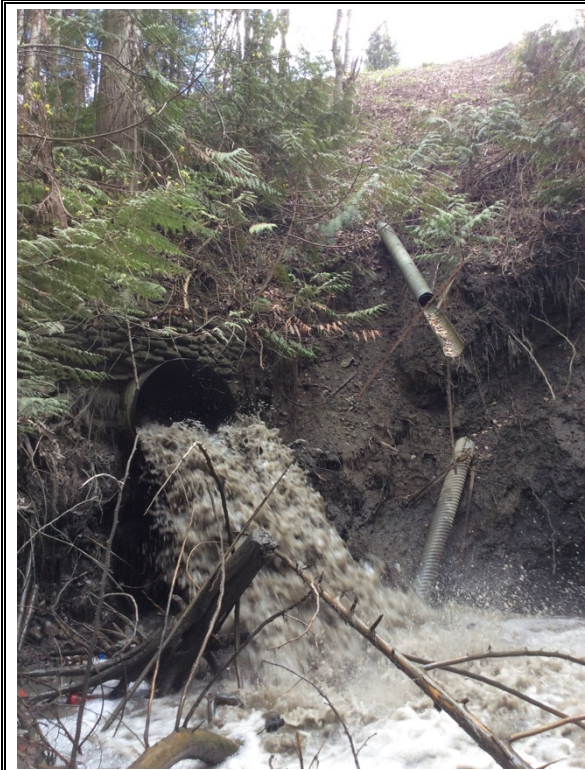
Photo 7 – View of culvert outlet (1200 mm diameter) in Highway 1. Note the scour in the embankment to the immediate right. [May 1, 2018]
