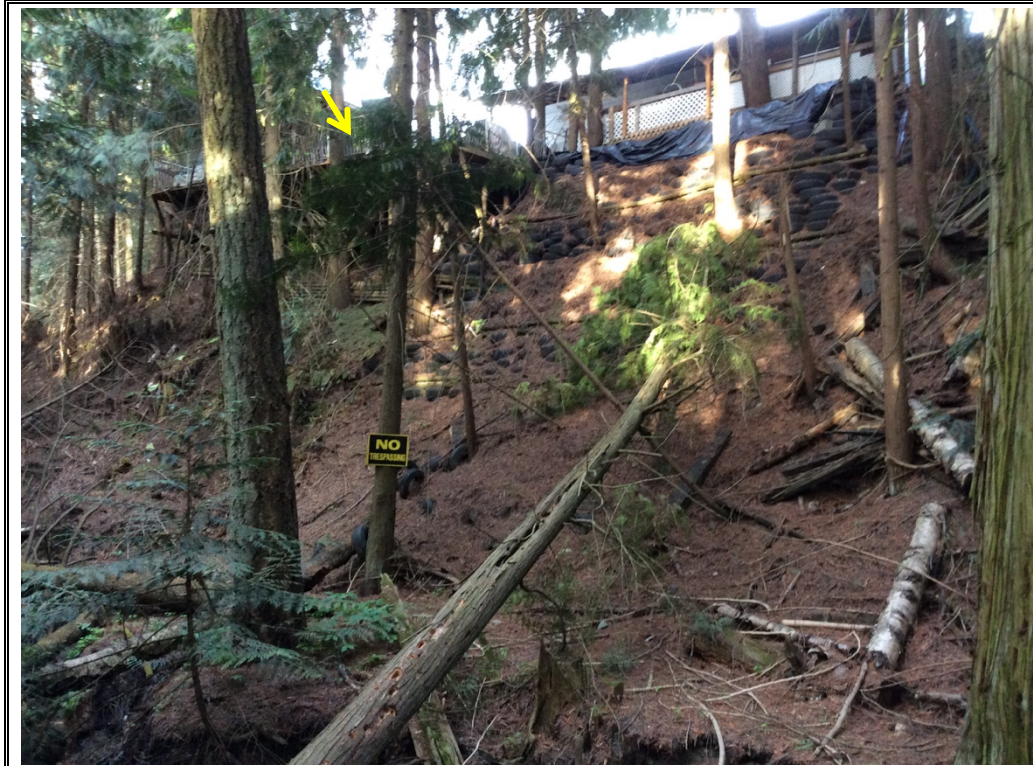
Photo 23 – 2825 Caen Road: view looking downstream (northeast) at the slope below the residence on this lot. Note the rubber tire retaining wall below the house. The elevated deck is shown with the arrow. [May 26, 2018]
