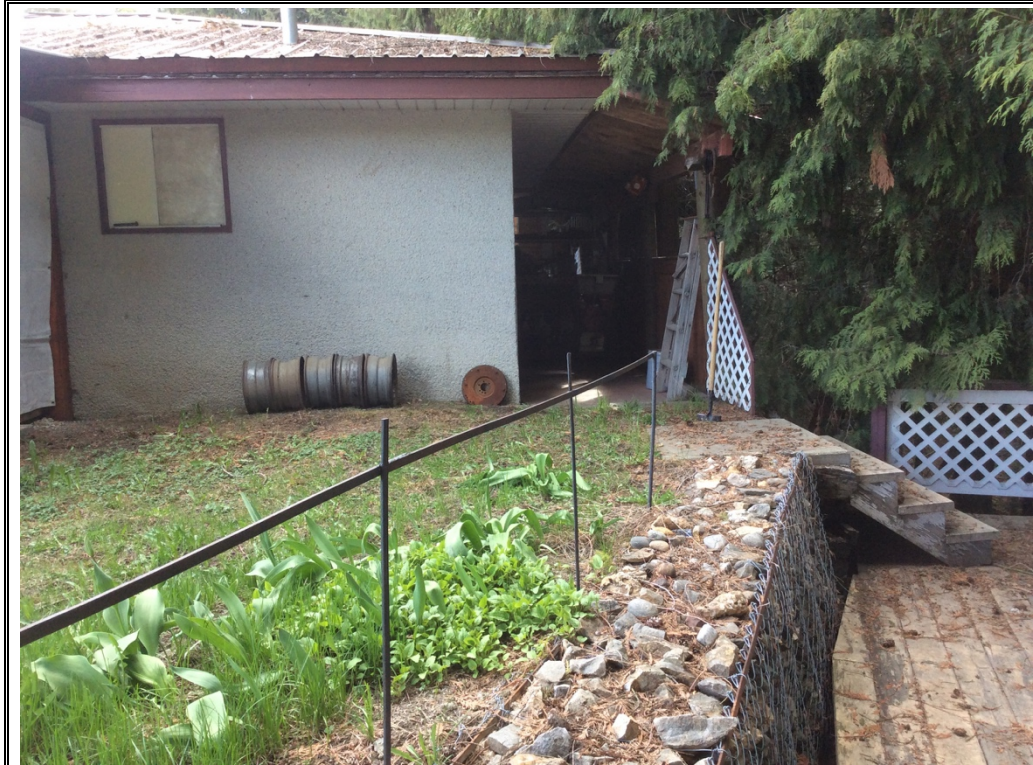
Photo 20 – 2823 Caen Road: view looking upstream (south) along the gully crest at the west side of the shop (~2 m setback). Note the fenced shed extends out to the crest (see Photo 21) and the gabion retaining wall and external patio deck in the lower right. [May 1, 2018]
