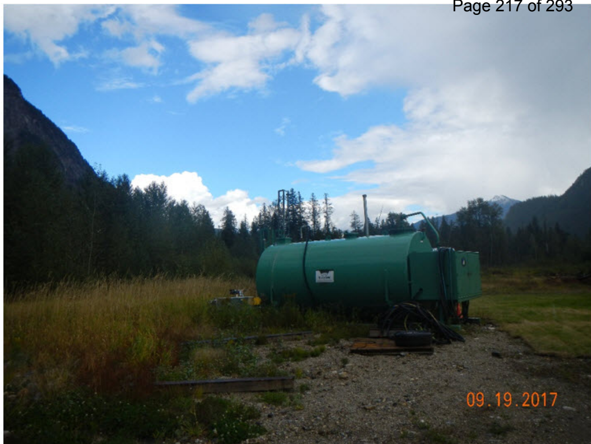
Fuel storage tank for helicopter refueling
