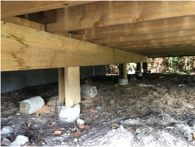
1-2x10 Post supporting ledger board & 2x10 joists, fastened to 4x4 post on 8" conc. columns
