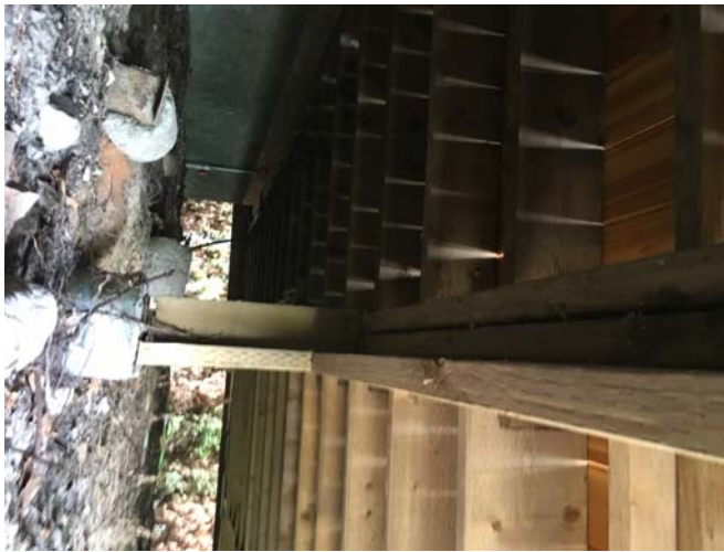
2 ply – 2 x 8 Beams supporting 2x 8 Joists
