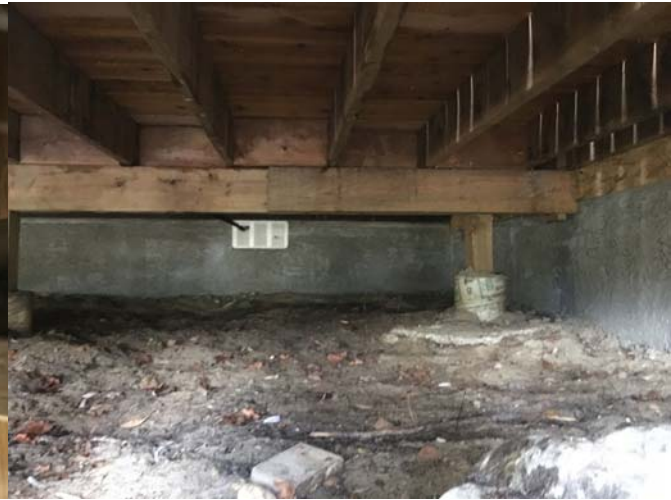
2 ply – 2 x 8 Beams supporting 2x 8 Joists with Scabbed on 2 x 8 to create a ledger board
