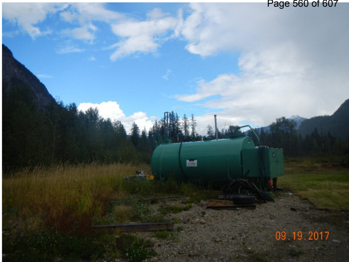
Fuel storage tank for helicopter refueling
