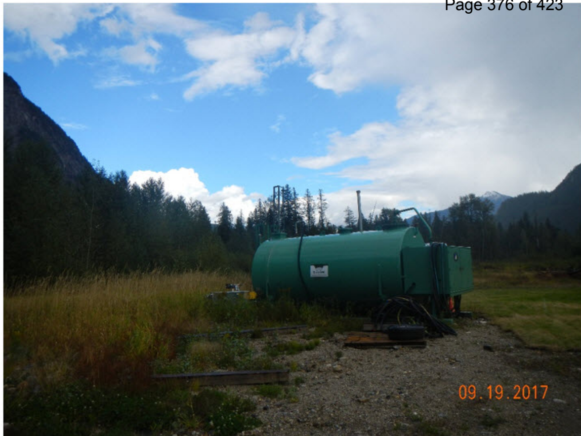
Fuel storage tank for helicopter refueling
