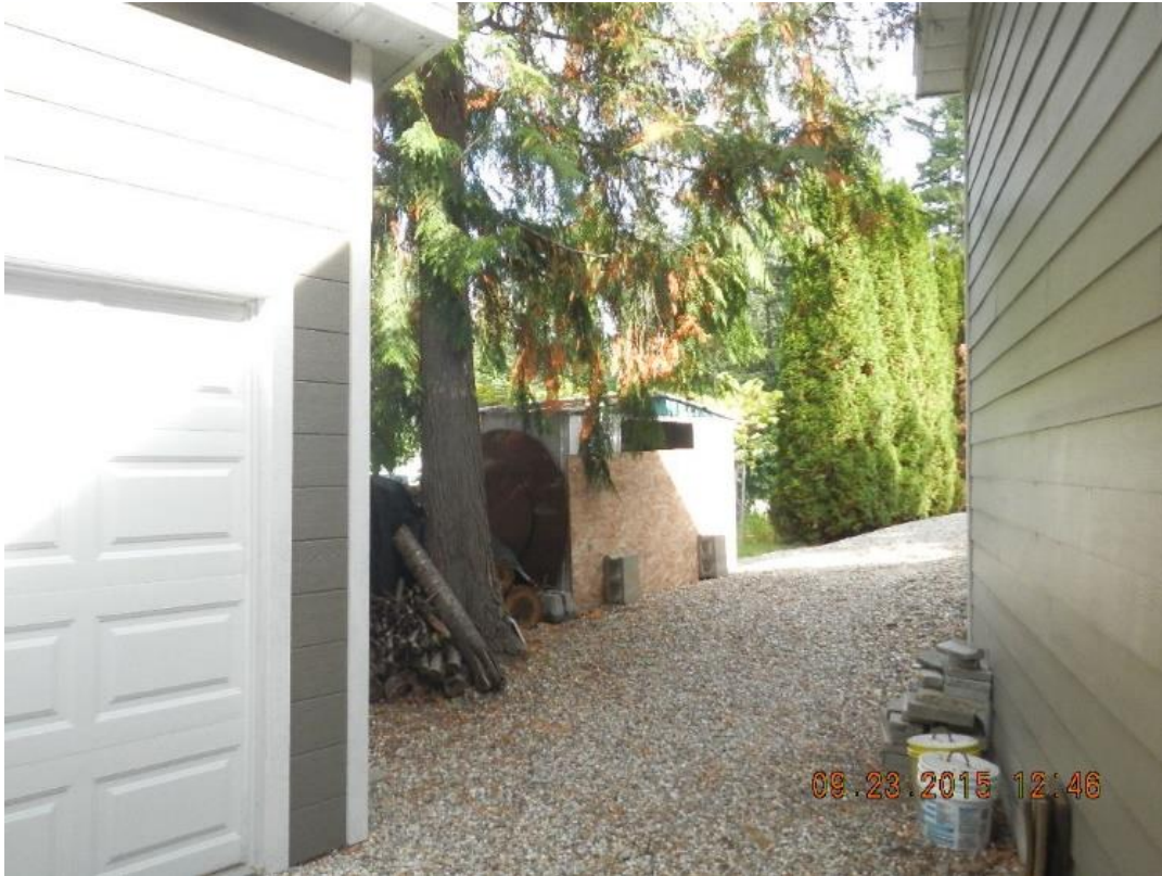
Left: shed on skids, Far center: shed on cinder blocks, Right: garage
