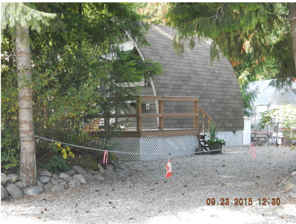
Accessory building/decommissioned bunkhouse
