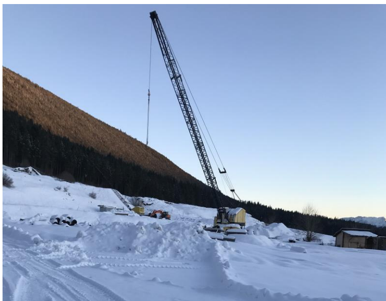
Photograph 1: Unused Log Yard
